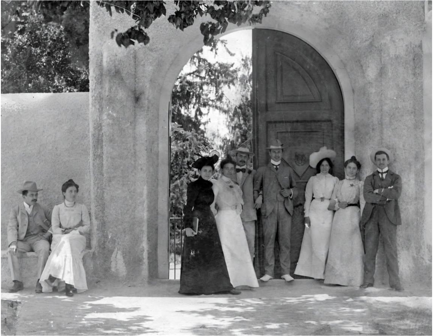
A Levantine house gateway on Genclik street, Bornova, sourced from the internet. This is the Edward Whittall house entrance, present view placed below for comparison. Identification of persons if possible would be appreciated.
