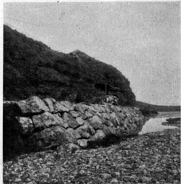
Fig. 11. Rock Block Protection.
