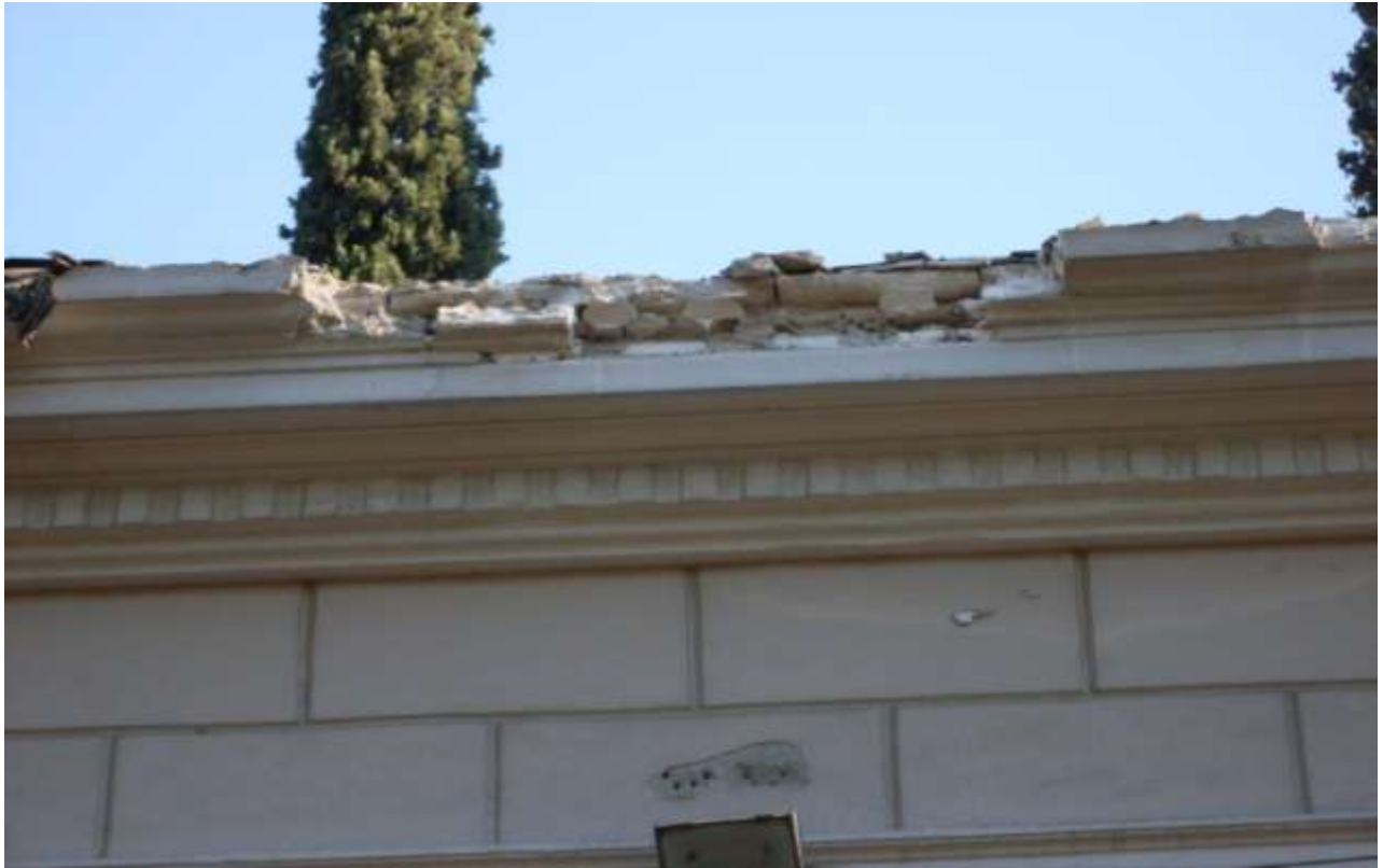
A close-up of the crumbling cornice before and after
