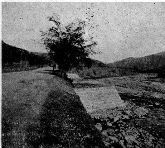
Fig. 13. Submersible Weirs Protecting Old Wall.
