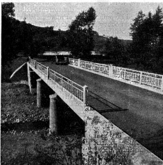
Fig. 19. Typical Concrete Bridge.
